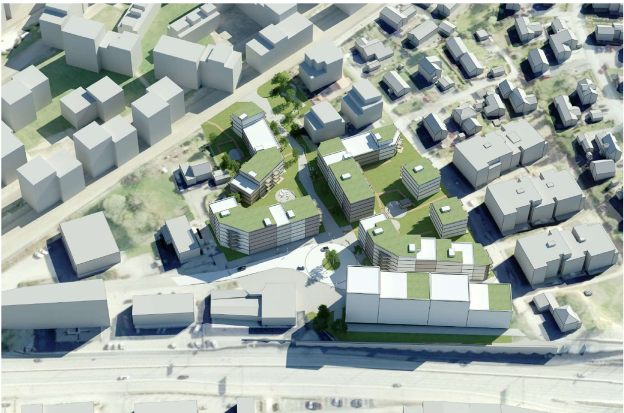
Gildheim is a residential project under development east of Trondheim city centre, with approximately 245 apartments.
